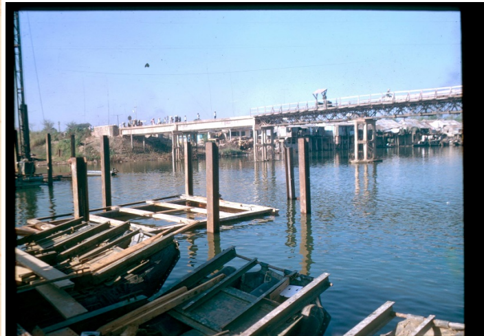
Dang Ha River Bridge Nov. 1969
